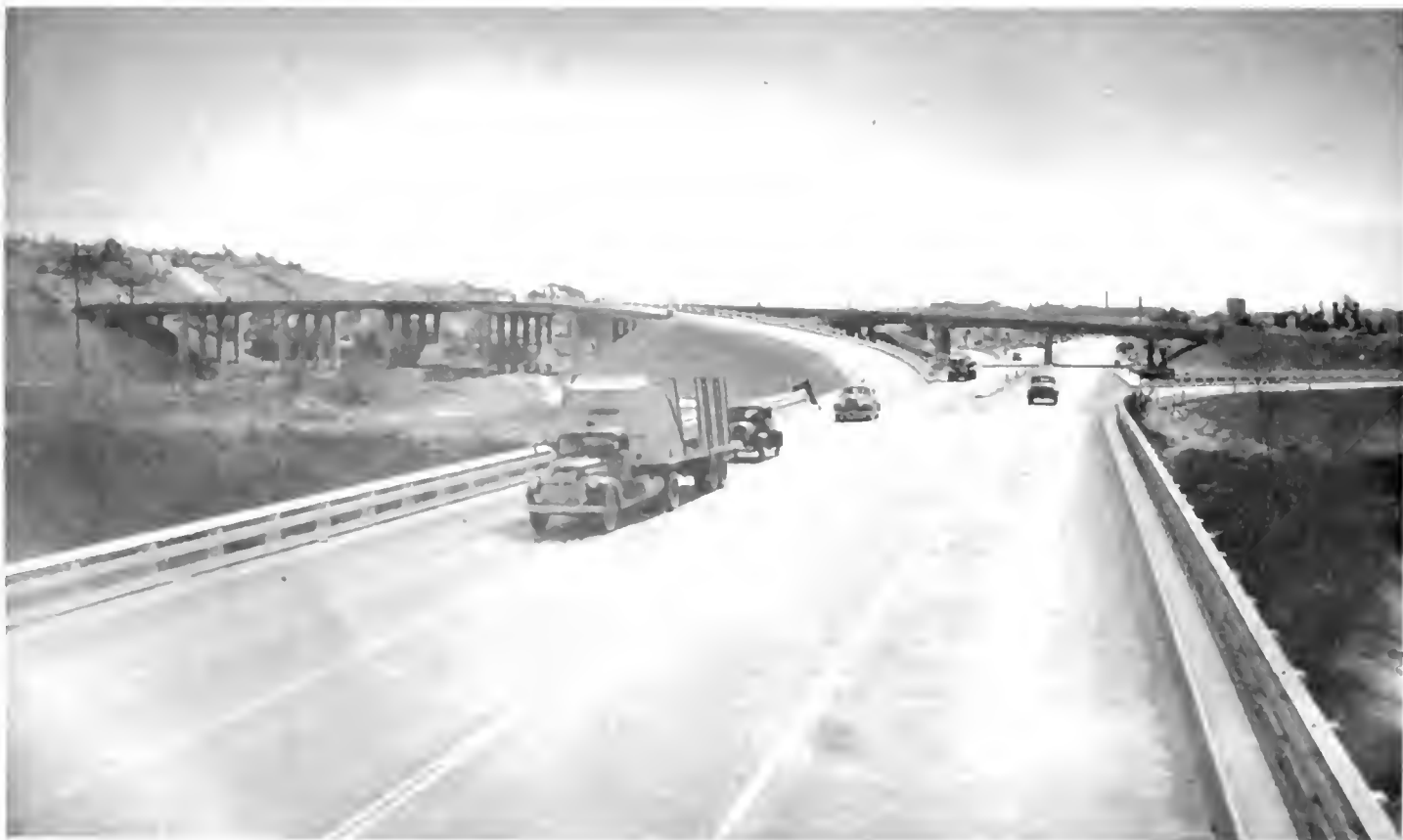
View of the Mission Valley Overpass in San Diego, looking south from the San Diego River
